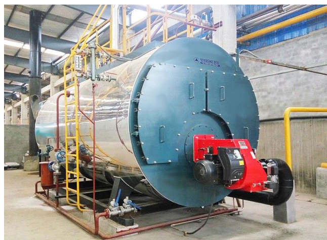
Figure 17. Fire Tube Steam Boiler Winketel (credit: Diemareng, CC BY-SA 4.0 < https://creativecommons.org/licenses/by-sa/4.0/ >, via Wikimedia Commons)
