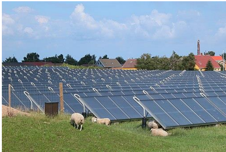
Figure 5. District heating using a solar thermal collector field of 18300 m 2 . Denmark, Marstal (credit: Erik Christensen, CC BY-SA 3.0 < https://creativecommons.org/licenses/by-sa/3.0/ >, via Wikimedia Commons)
