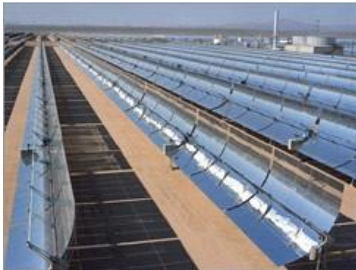
Figure 4. Medium Temperature parabolic trough arrays (credit: ArséniureDeGallium, Public domain, via Wikimedia Commons)
