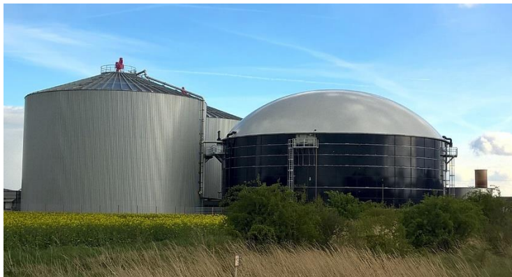
Figure 8. Biodigester CSTR (Continuous-flow Stirred Tank Reactor) for biogas production (credit: geraldK (pixabay.com))
