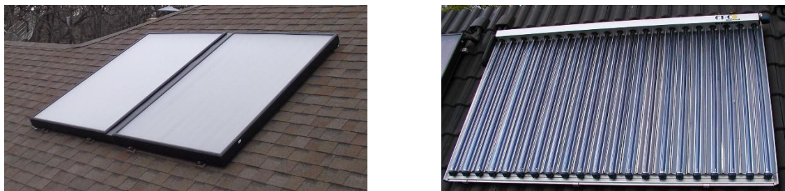
Figure 4. Flat tube collector (left) and evacuated tube collector (right)
